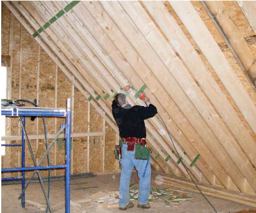
Figure 7. Ties made from Zip sheathing scraps connect 2x3 extensions to the 2x10 rafters to create a 14-inch-deep insulation cavity (left). Blocking between rafters is fully caulked around the edges to prevent air movement and moisture migration through the cellulose insulation (below left). Gable walls are framed with double top plates in lieu of end rafters, breaking conductivity through framing members and creating an unobstructed insulation cavity (below).
