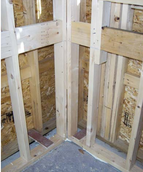
Figure 5. The bottom plates of the inside walls sit directly atop the slab's perimeter insulation, preventing a direct mechanical connection to the concrete. To hold the walls parallel to the exterior walls, the author used plywood standoffs and sealed beneath the plates with expanding foam (left). Single-stud corners reduce thermal bridging and allow fuller insulation coverage. Wall plates running parallel to the ceiling joists are nailed to 1x3 ceiling strapping, eliminating redundant framing (above).
