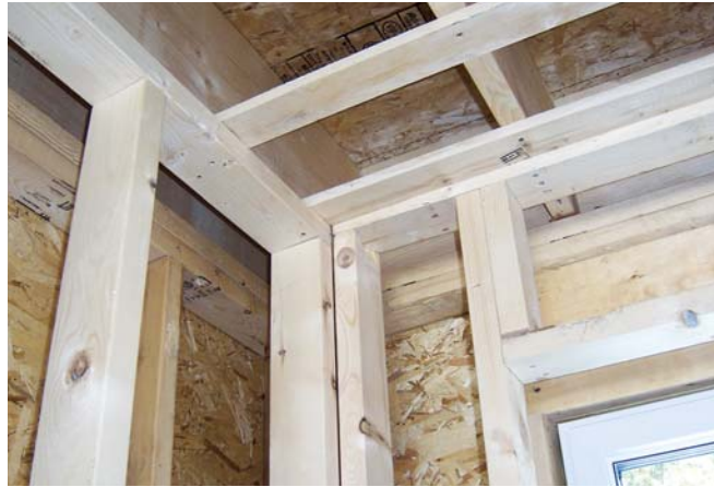
Figure 5. The bottom plates of the inside walls sit directly atop the slab's perimeter insulation, preventing a direct mechanical connection to the concrete. To hold the walls parallel to the exterior walls, the author used plywood standoffs and sealed beneath the plates with expanding foam (left). Single-stud corners reduce thermal bridging and allow fuller insulation coverage. Wall plates running parallel to the ceiling joists are nailed to 1x3 ceiling strapping, eliminating redundant framing (above).
