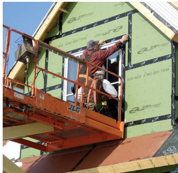
Figure 2. With the seams taped, Zip System sheathing provides a water-resistant air barrier under the siding.
