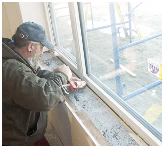
Figure 11. Condensation on a very cold day during construction indicated gaps around this window that were not revealed during blower-door testing. The author stripped back the drywall returns and caulked around the jambs.
