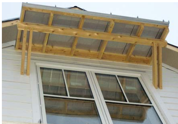
Figure 4. Fixed awnings shade south-facing windows from high summer sun while allowing lower-angled solar gain during the winter months.
