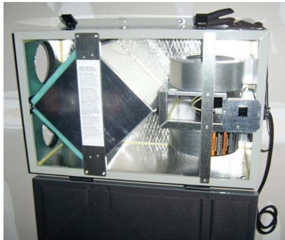
Figure 10. An energy recovery ventilator (ERV) provides whole-house ventilation while capturing heat held in humid indoor air and transferring it to the incoming fresh air.
